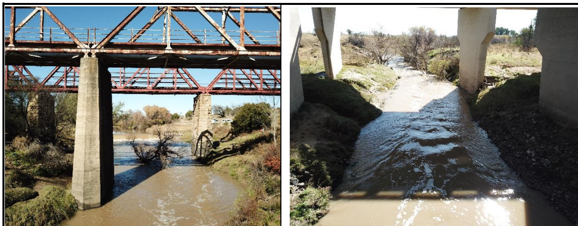
Figure 7-20: Site photographs of the Upper Modder EWR site
