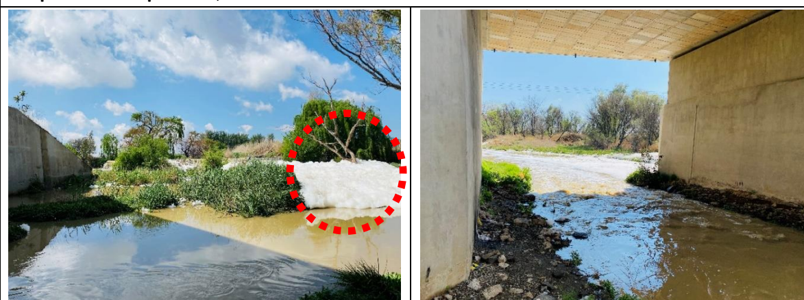
Figure 9-12: Site photographs of the Renoster field verification site (The red dotted line indicates the foam, indicative of raw sewage)
