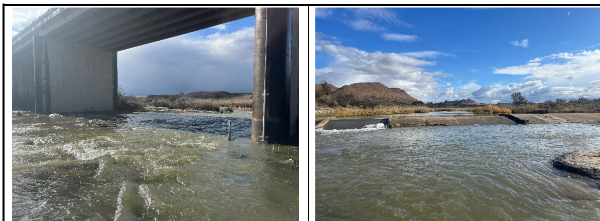
Figure 7-14: Site photographs of the Seekoei EWR site
